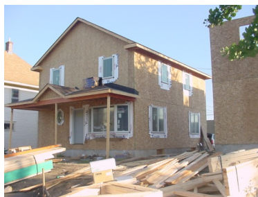
671 Aurora under construction September 2005
