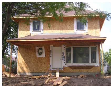
895 Central Avenue Currently under construction
