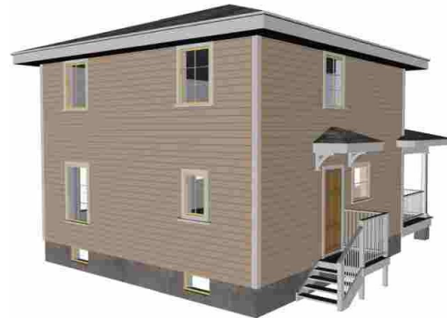
NORTH /WEST VIEW
