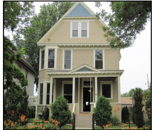
One of the MCASA houses
